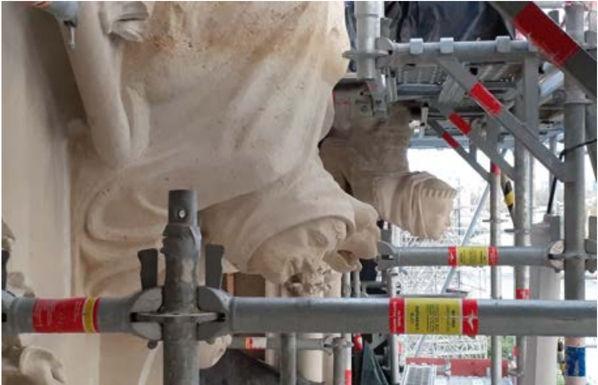
Installation of the sculptures copied from the former ones – South gable
