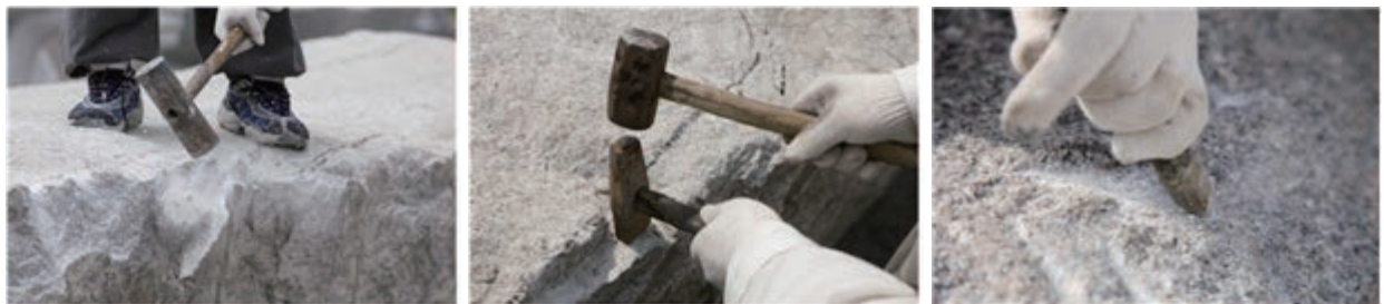
Figure 3: Various stone processing (knobbing / chiseling / boasted work)
