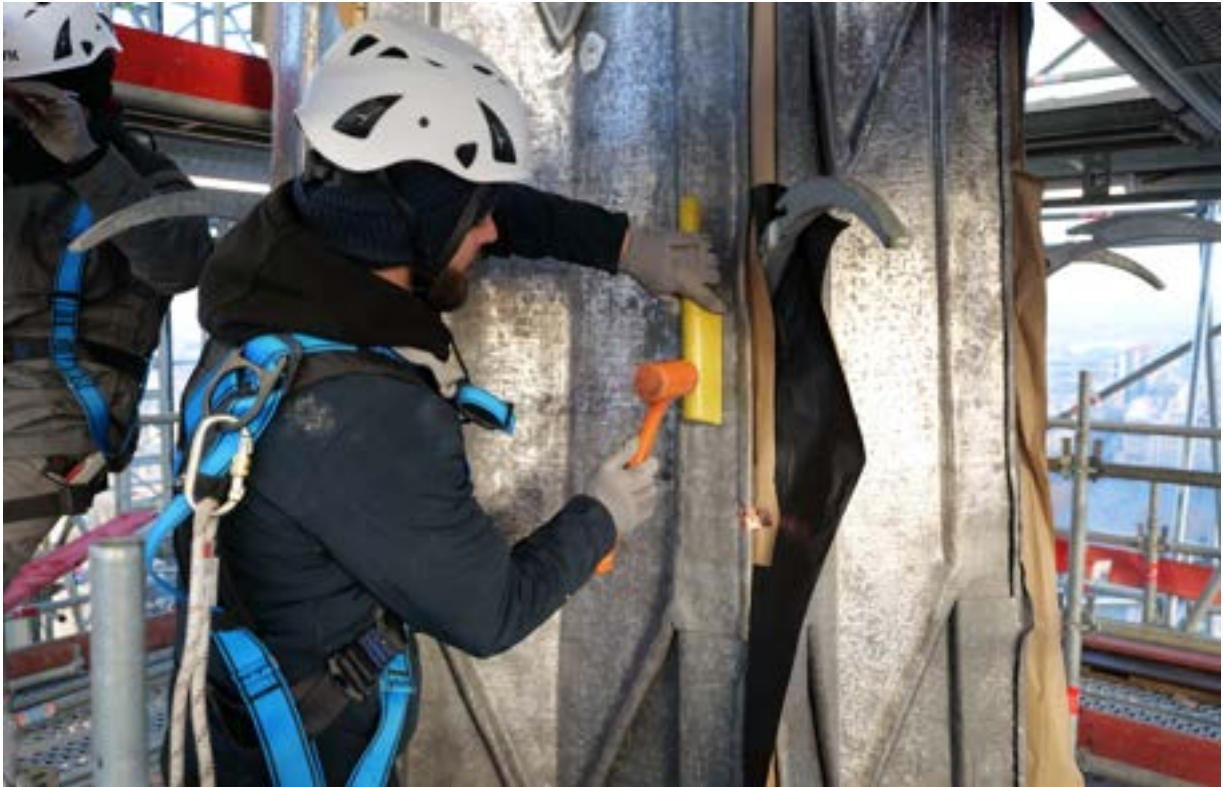
Installation of the lead cover on the spire needle
