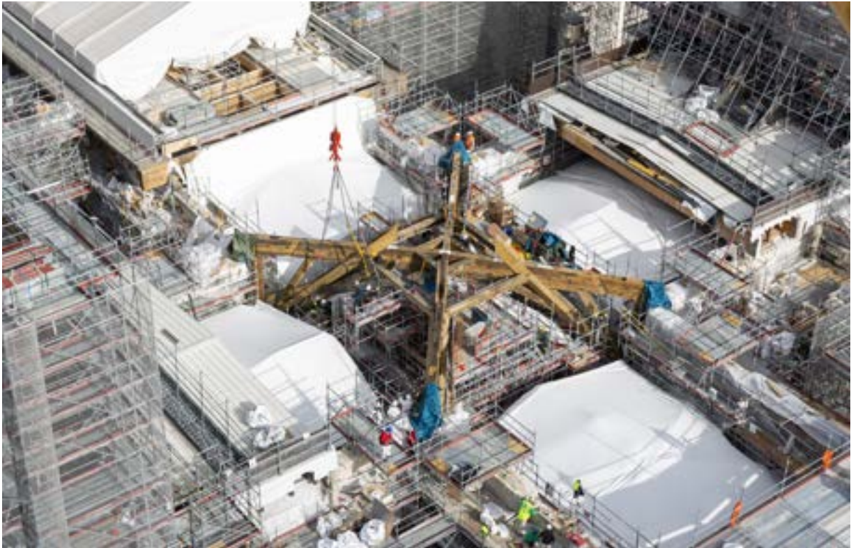
Final assembly of the base of the spire at the crossing transept
