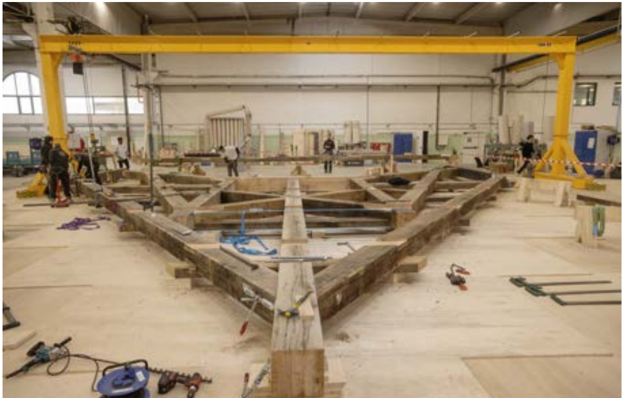
Assembly test of the base of the spire in workshop
