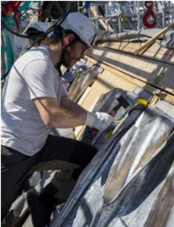
Installation of the lead cover on the nave and the choir
