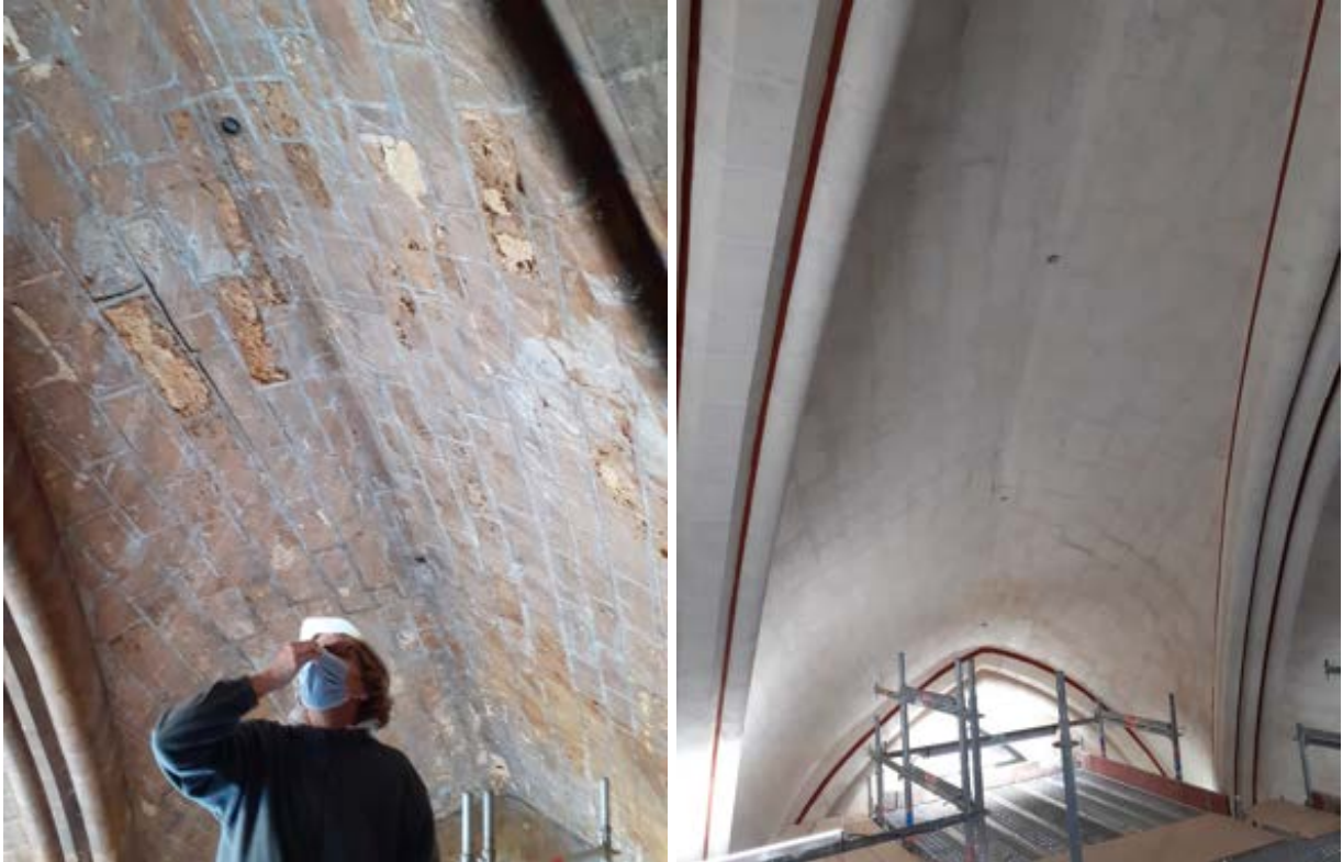
Restoration of the vaults of the south transept – before/after
