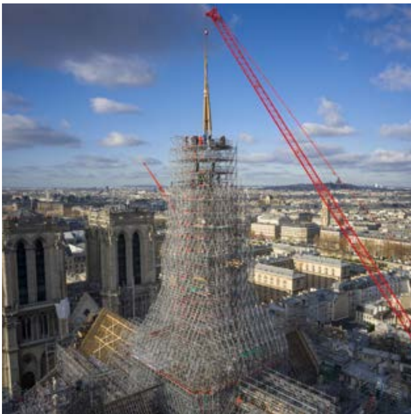
Completion of the spire framework
