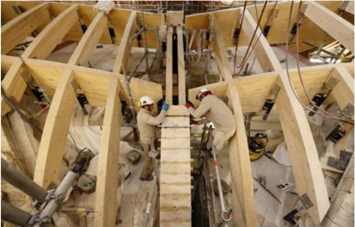
Rebuilding of the collapsed vaults
